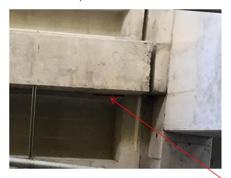
AREA ABOUT 3' LONG WHERE REBAR IS EXPOSED. OVERHEAD REPAIR.
